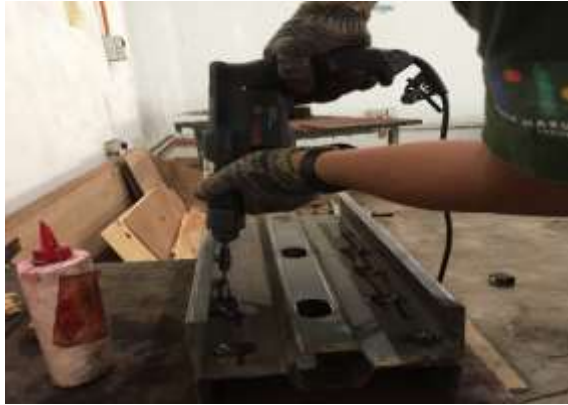
Figure 3.9 Drilling for Built-up Sigma section
