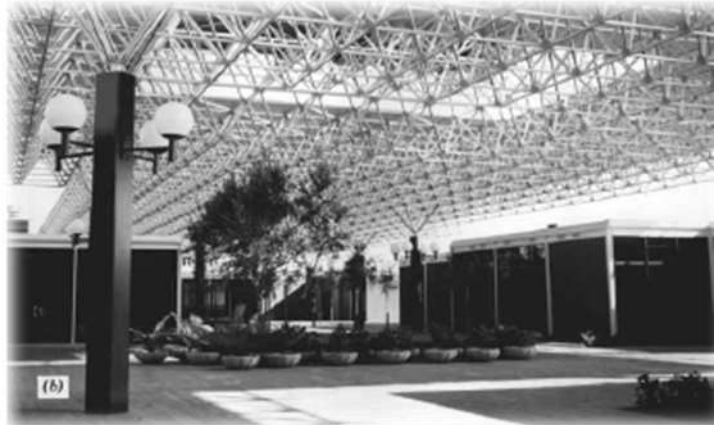
Figure 2.3 Cold-formed steel sections used in space frames
