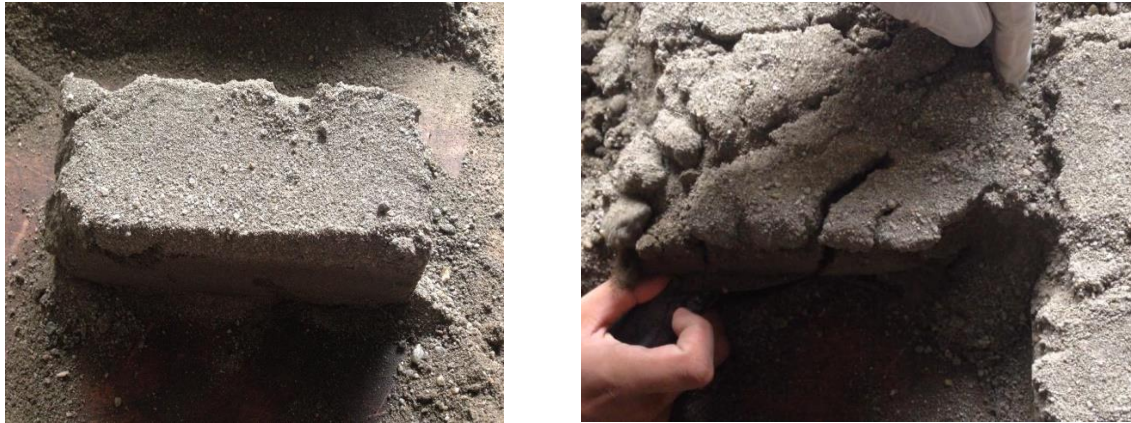
Figure 4.3 Condition of sand brick with 5% replacement after taking out from the mould
