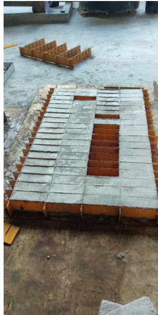
Figure 3.7 Formwork and Moulded Cement Sand Brick In the Formwork
