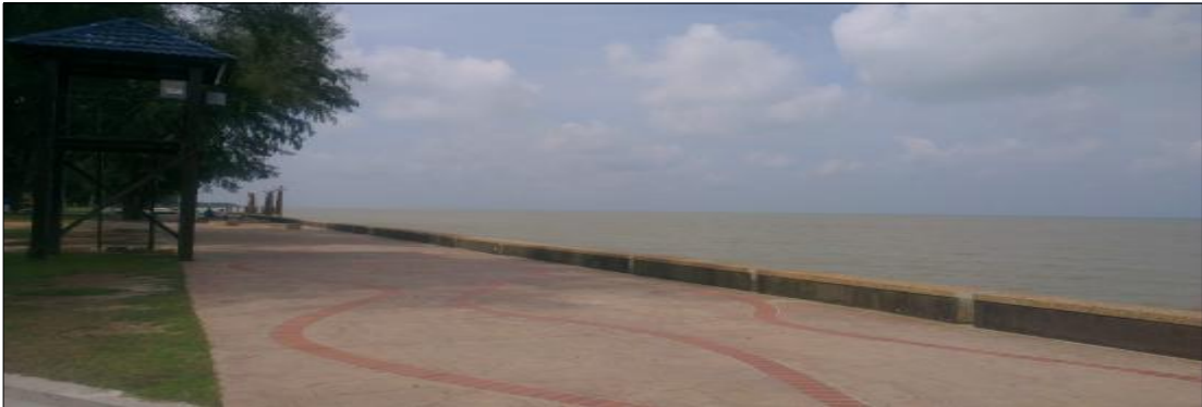
Figure 1.3 Example of Retaining Wall at Pantai Morib, Selangor
