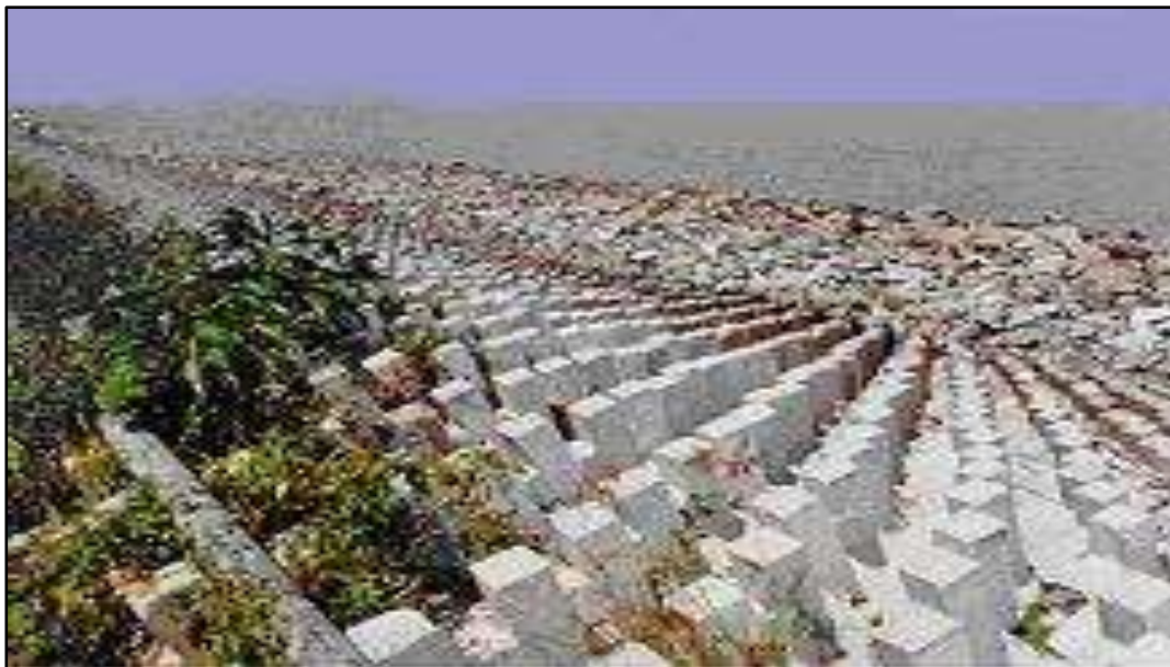
Figure 4.10 Example of Existing SAUH Revetment at Sungai Burung, Selangor
