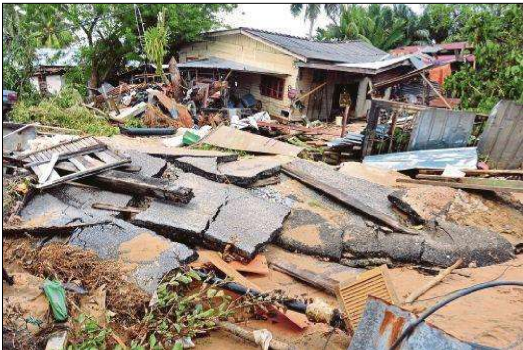
Figure 1.5 The Damage Happened due to Sea Level Rise at Tumpat, Kelantan
