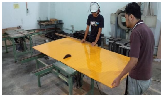
Figure 3.10 Cut the plywood following the right size to make formwork
