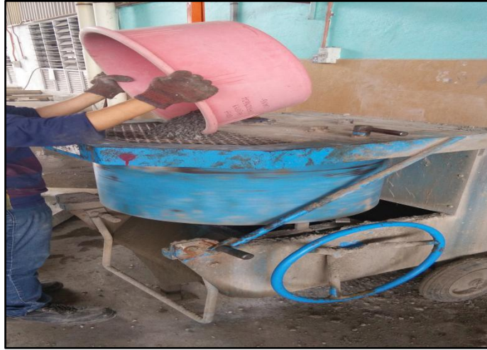
Figure 3. 11 Pouring Material into concrete pan mixer
