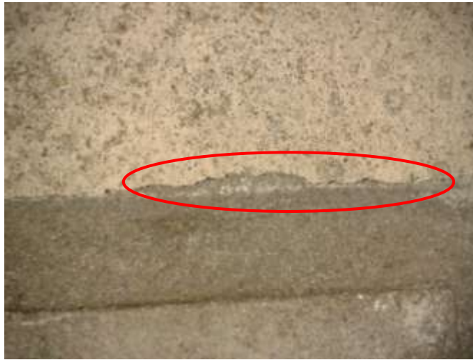
Figure 4.17: Leakage from cavity mould.
