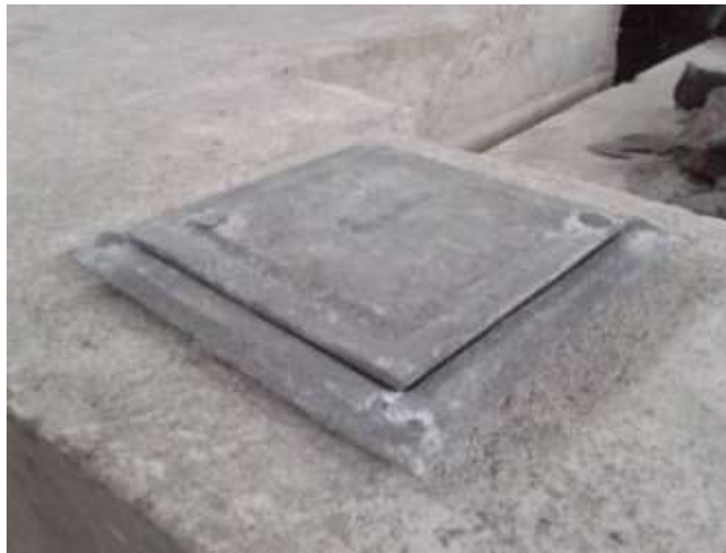
Figure 4.18: Have gap between hole cover and frame.
