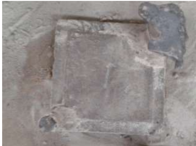
Figure 4.3: After casting the hole cover, top view.
