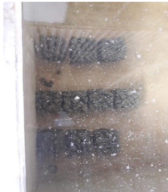
Figure 3.15 Curing for pervious concrete
