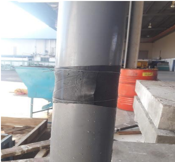
Figure 3.22 Outside view for where the PC is placed
