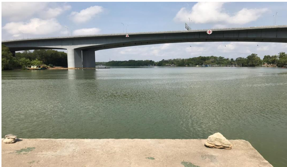
Figure 1.2 Bukit Kuang Bridge, Kemaman, Terengganu
