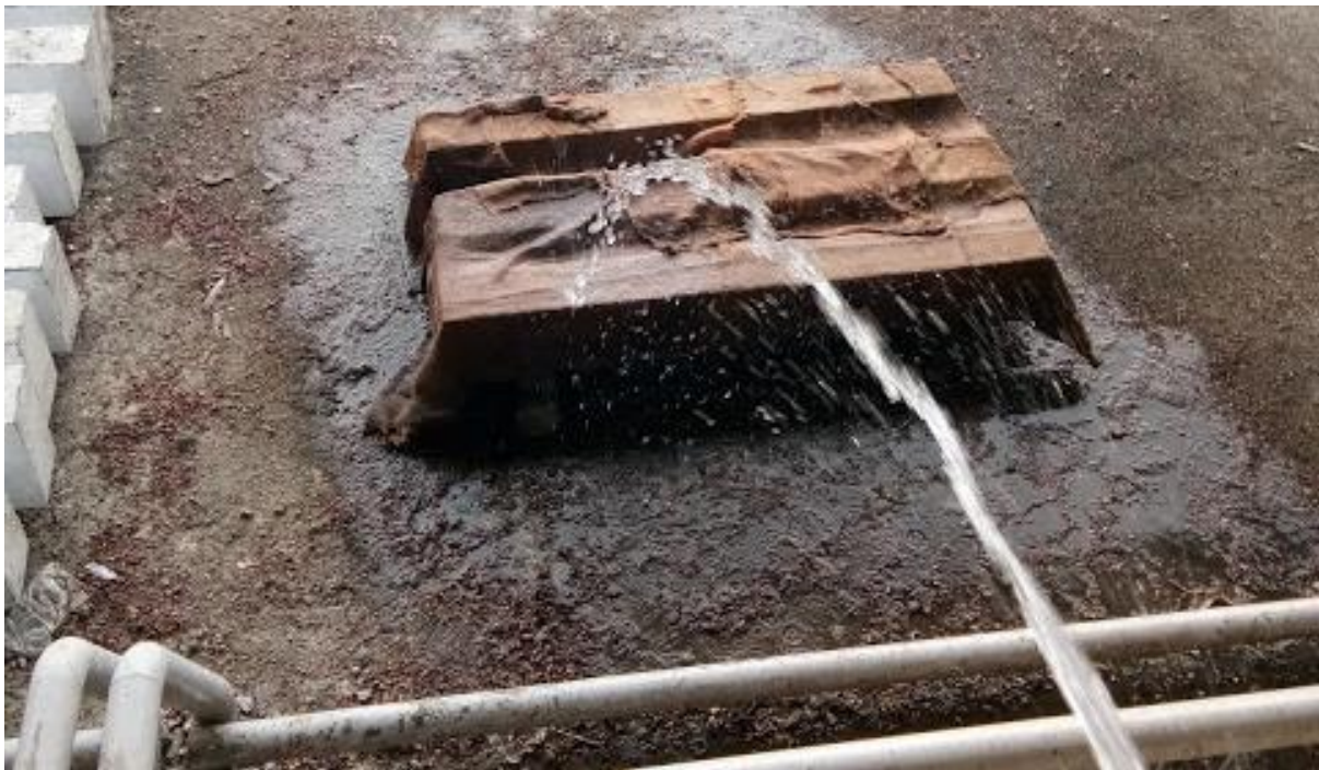
Figure 3.9: Curing process.
