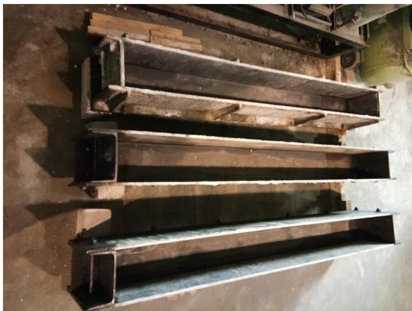
Figure 3.2: Formwork of the beams.
