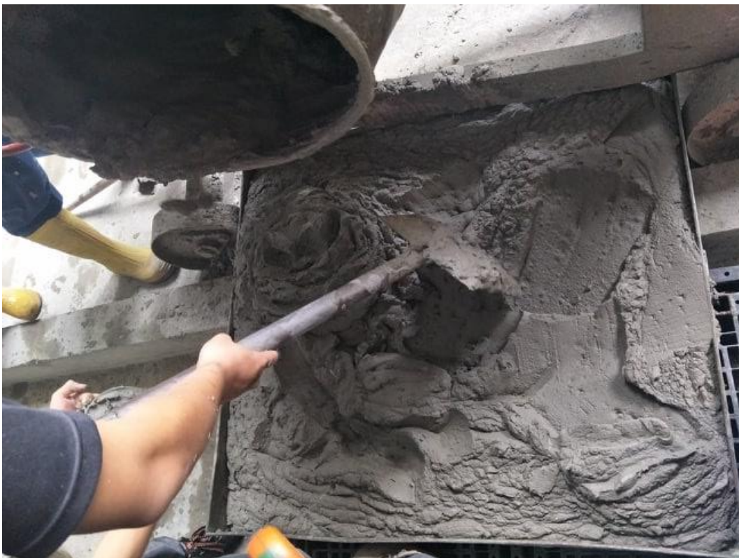
Figure 3.7: Fresh foamed concrete right after mix.
