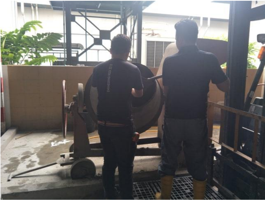
Figure 3.6: Mixing foamed concrete materials.
