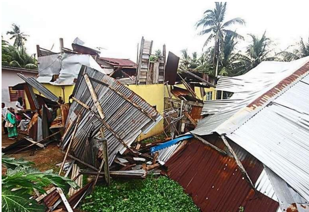
Figure 1.1: Damages caused by the tornado in Kampung Sungai Nonang
