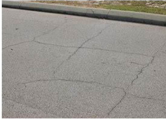
Figure 6 : Block Cracking
