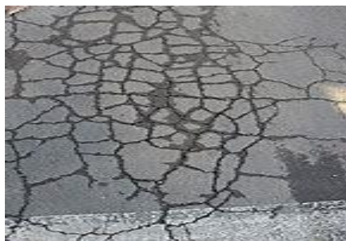
Figure 3 : Fatigue Cracking
