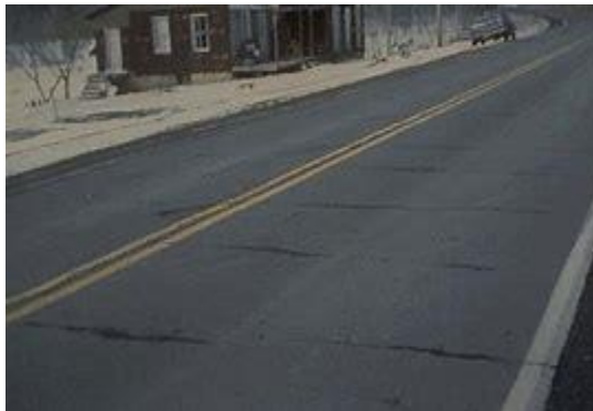
Figure 5 : Transverse Cracking
