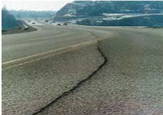
Figure 4 : Longitudinal Cracking
