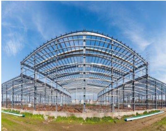
(a) Commercial building
