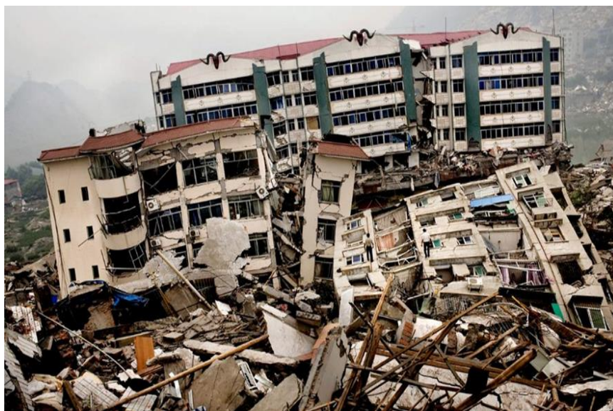
Figure 2.1 Damages of residential building because of the earthquake disaster
