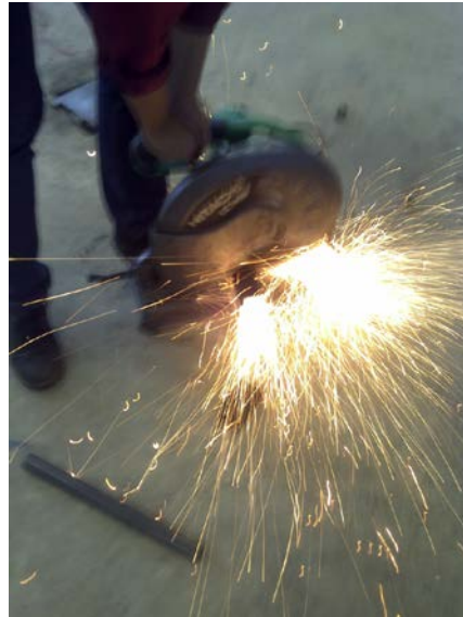
Figure 3.2: Cutting material using disc cutter
