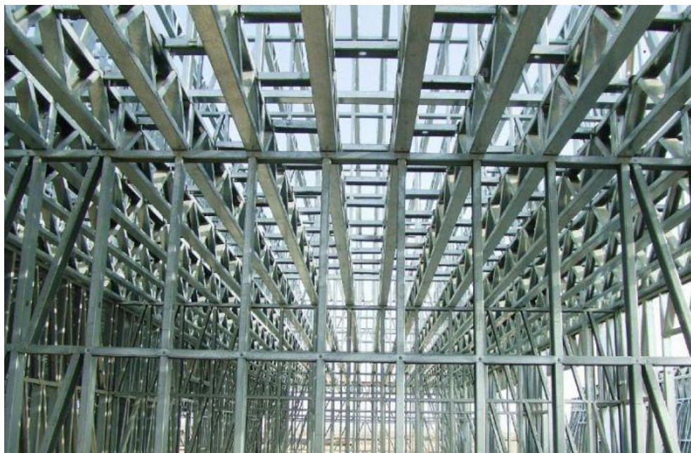
Figure 1.2 Cold-formed steel framing
