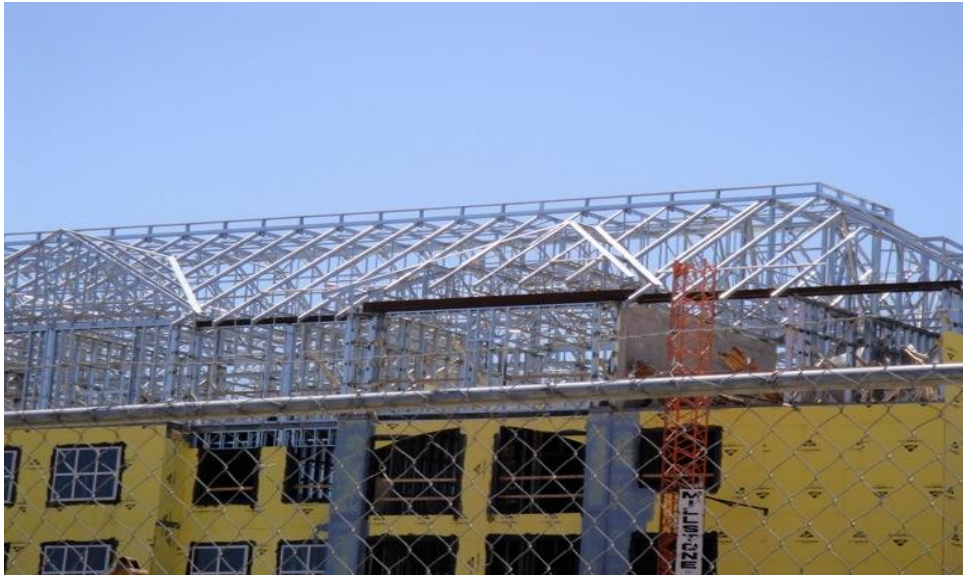
Figure 2.2 Roof system using cold-formed
