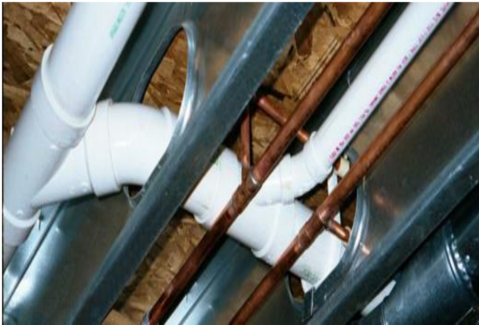
Figure 2.3 CFS with opening to accommodate piping system
