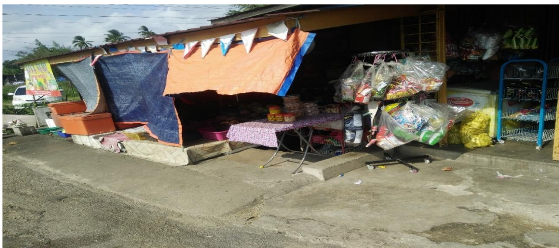
Figure 4.6 One level building
