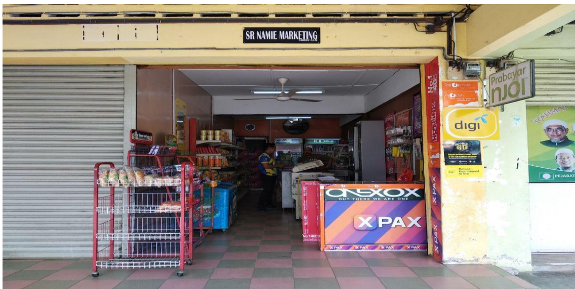
Figure 4.5 One level building
