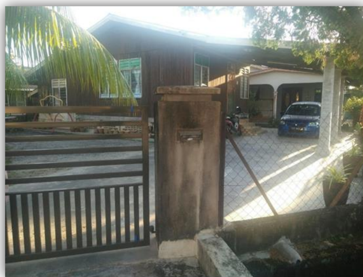
Figure 4.7 Single storey house's construct with timber at Sungai Isap
