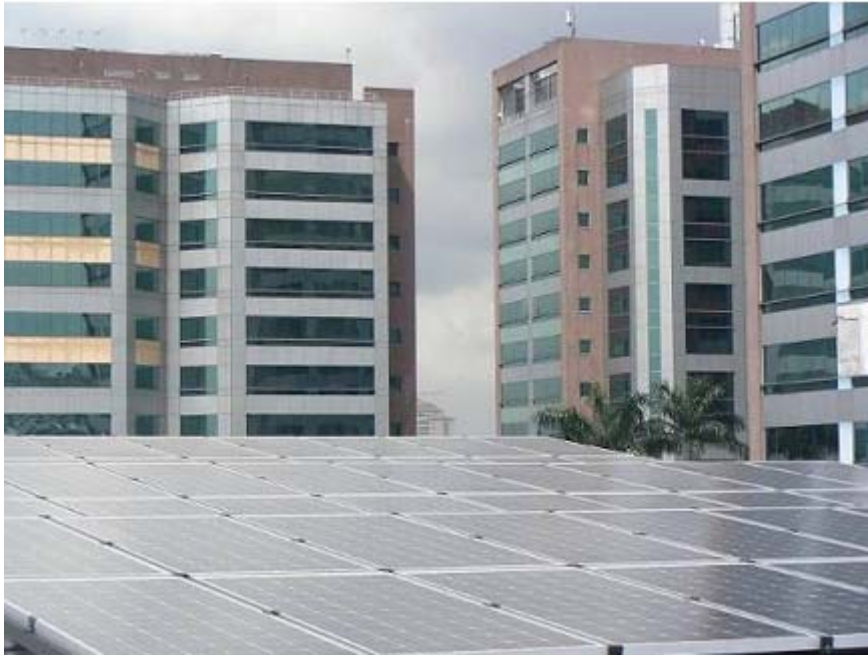
9.9 kWp Damansara Utama (Selangor) BIPV in 2007
