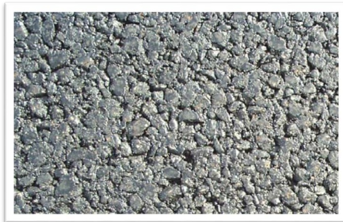
Figure 2.12: Typical Stone Mastic Asphalt surface
