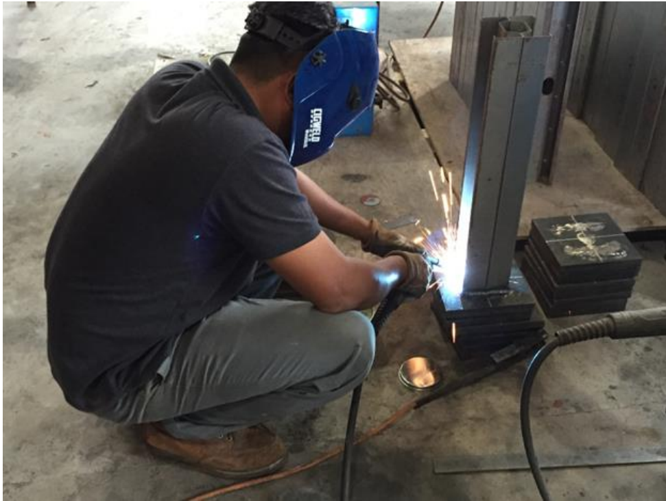
Figure 3.8 Technician welding the specimen
