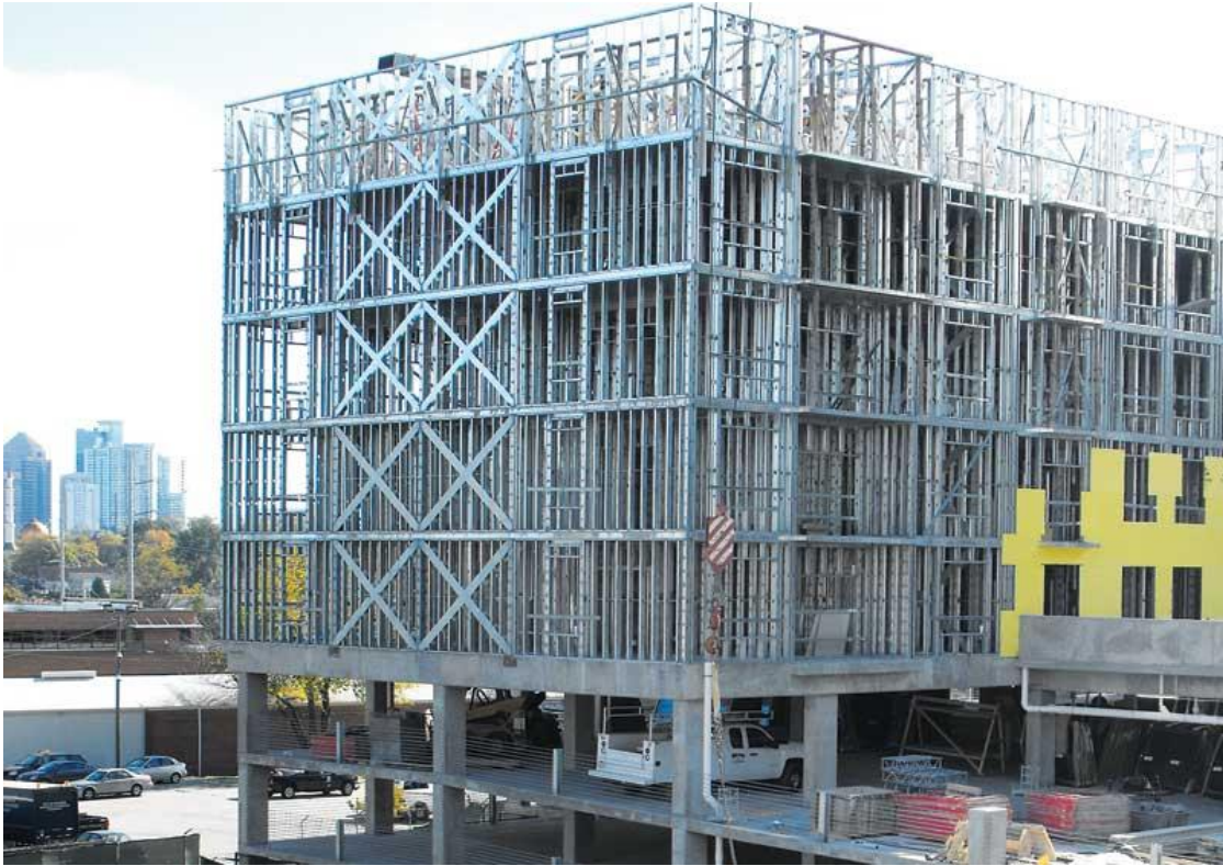
Figure 1.1 Building composed entirely of cold-formed steel sections
