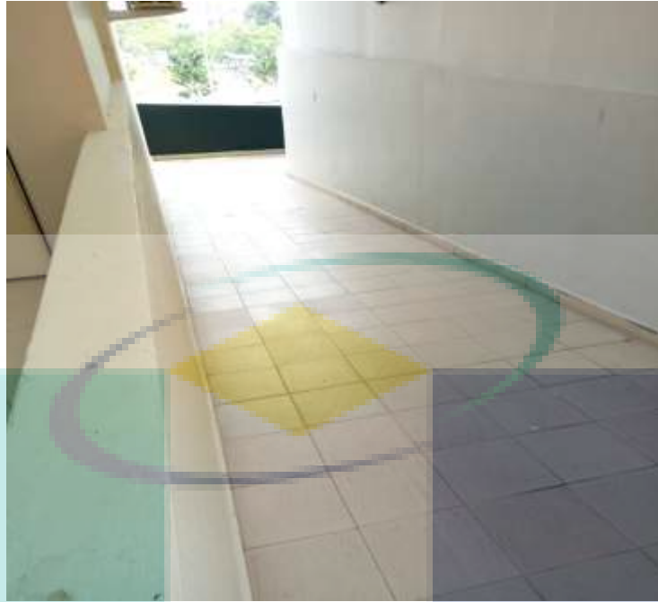
Figure 3.23 Slope condition for wheelchair at UMP
