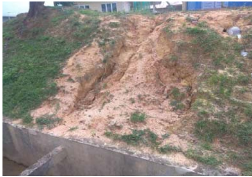
Figure 1.1: Shows that the soil is badly eroded
