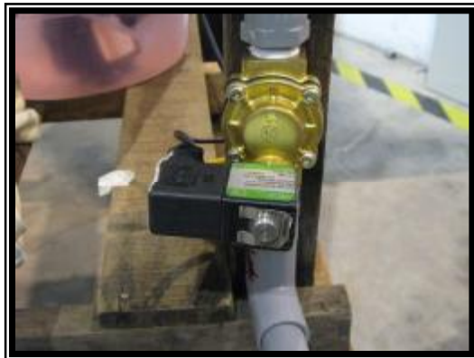
FIGURE 4.15 : Switcher Valve After Installation
