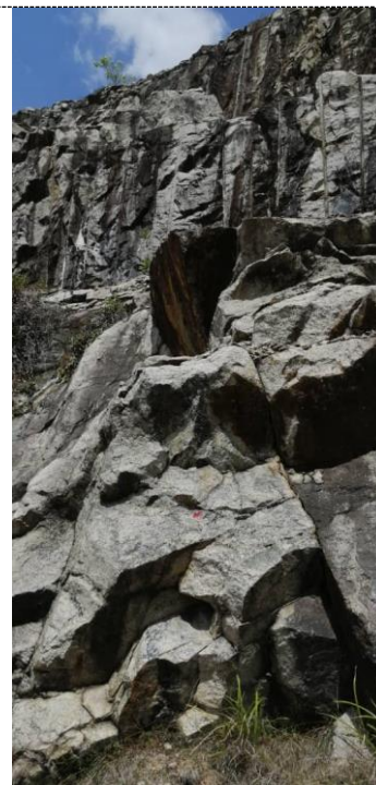
Figure 6. View of potential wedge failure on the slope (Panel 4)
