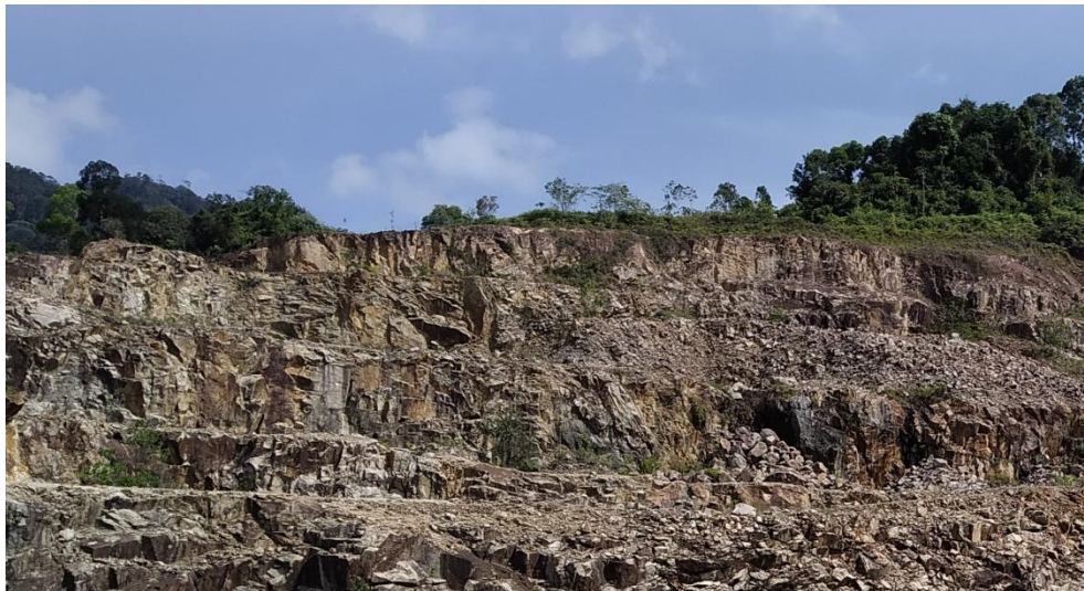
Figure 1. View of the exposed cut slope at Sri Jaya
