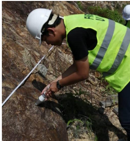
Figure 7. Using the Schmidt rebound hammer in the field
