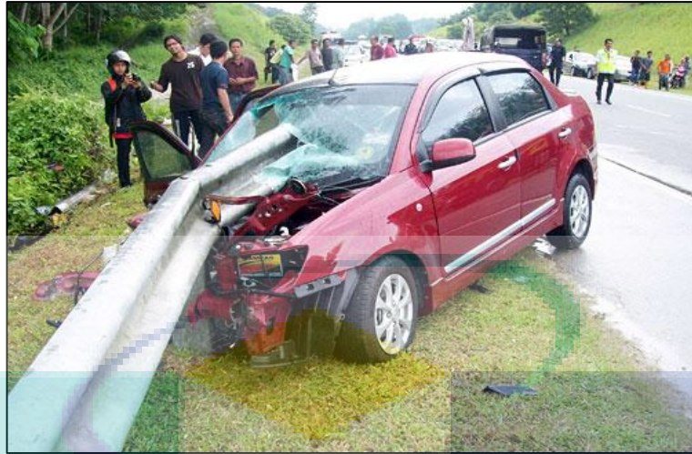
Figure 4.55 A metal barrier penetrated into skidding car causing 4 died at KM 73 Kuala Kangsar Road, Gerik, Perak
