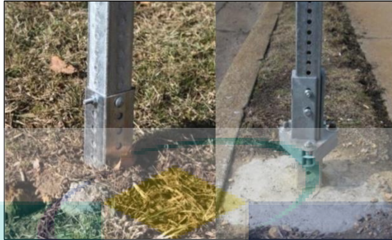
Figure 2.11 U-channel post, sleeve assemblies as the base (left) or slip couplings (right)
