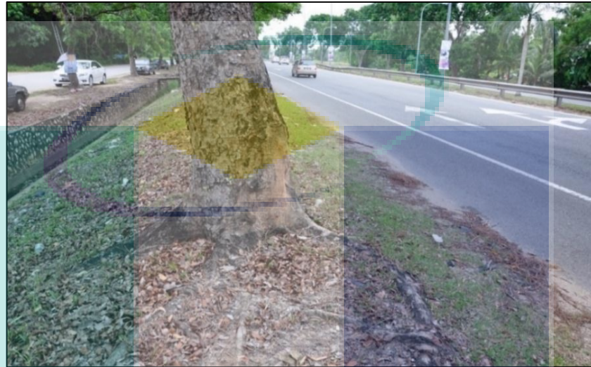
Figure 4.28 A tree with 490 mm diameter is located 3.8 metres away from the travel lane located at KM 5 Gambang-Kuantan road, Pahang. The tree root spans about 1 metre towards the travel lane
