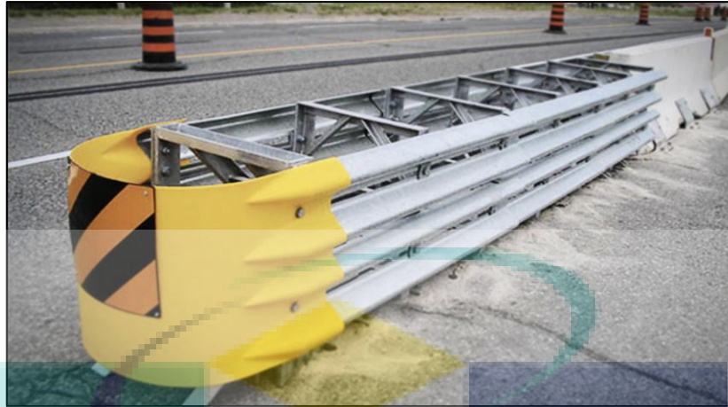
Figure 2.3 Safety barrier with blunt end with crash cushion
