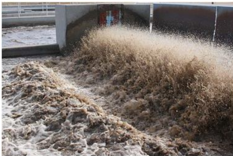
Figure 2.1 Activated sludge are aerating properly (Durbin M., 2008)
