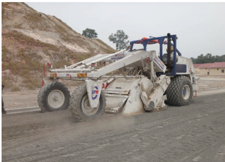
Fig. 3 Dry mixing process using stabiliser machine
