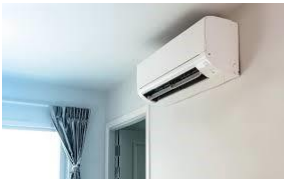
Figure 1: Wall-mounted split unit type air conditioner
