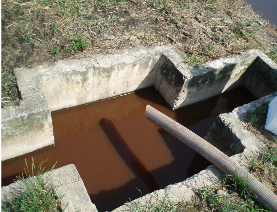
Figure 4.5: Recycle path to balance microbe concentration
