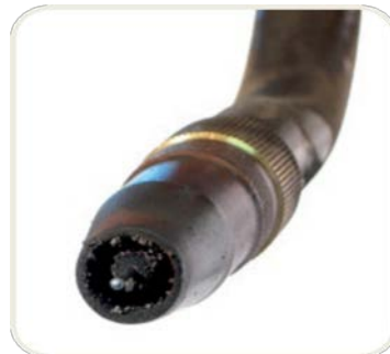
Figure3.3: Corrosion (Rinaldi, E. 1979)
