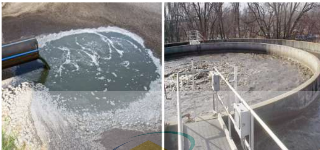
Figure 2.2 Petrochemical wastewater treatment plant
