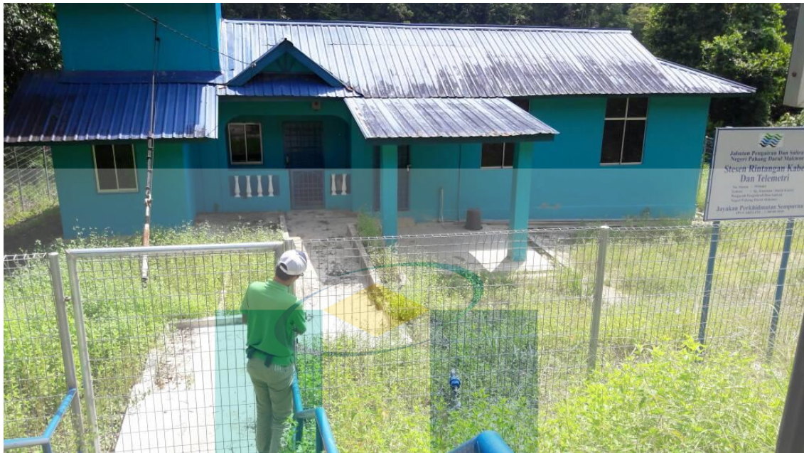
Figure A3 The Telemetry Station at Bukit Kenau
