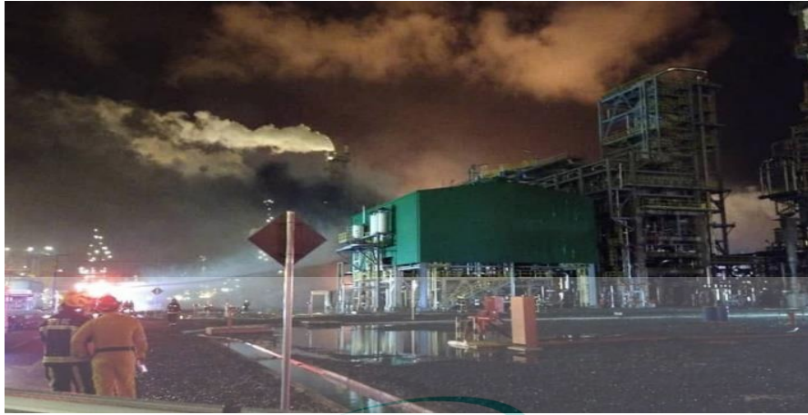
Figure 1.1: Fire and Explosion Incident at RAPID Pengerang
