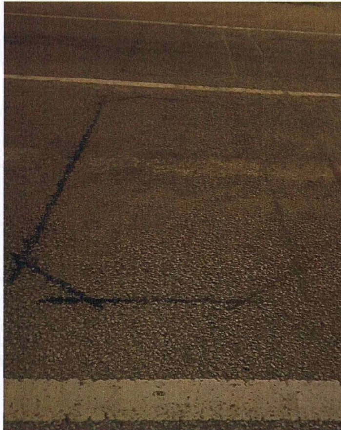
Figure 3-2: Loops under the road
