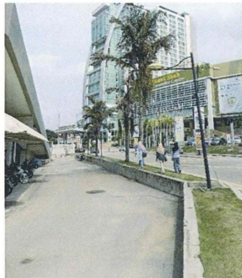
Figure 4.32 Site area 2 in Stretch 3 (C-D).
