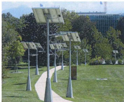
Figure 2.2 Solar-powered LED lighting along the walkway.
