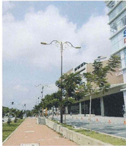
Figure 4.31 Site area 1 in Stretch 3 (C-D).
