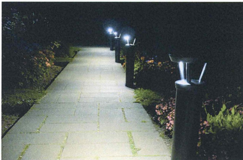
Figure 2.3 Light bollards illuminating the pedestrian walkway.
