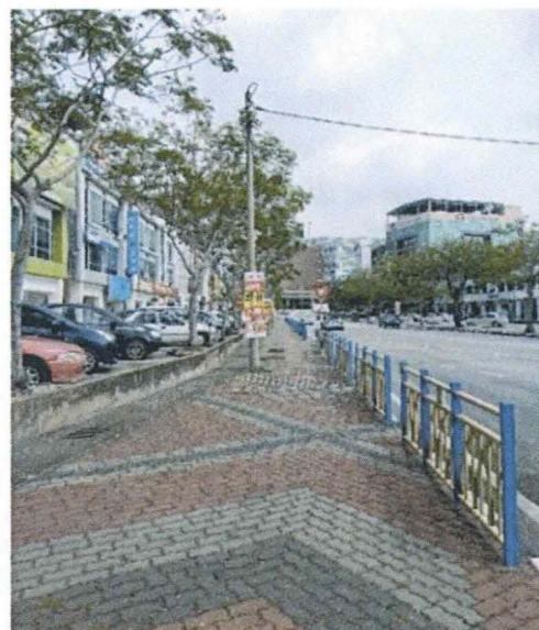
Figure 4.29 Site area 2 in Stretch 2 (B-C).
