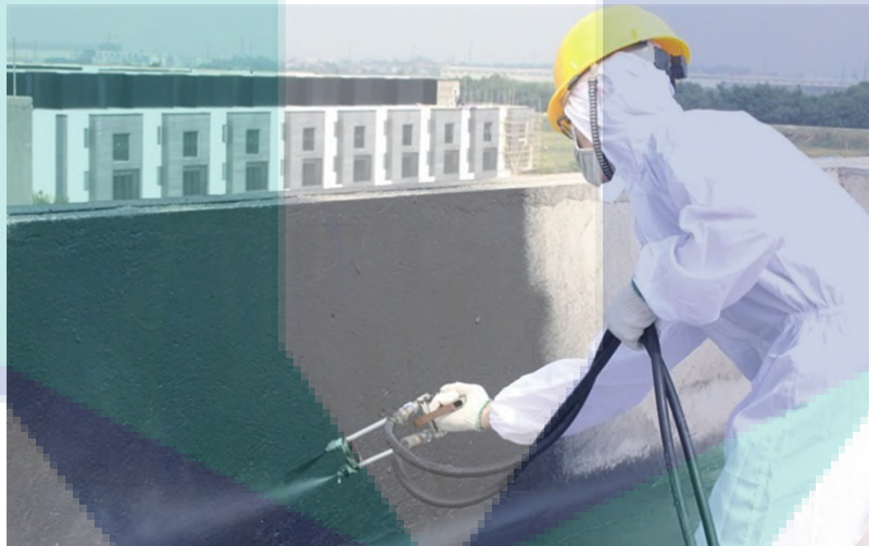
Figure 2.4: The Application of EMB as Wall Insulator
