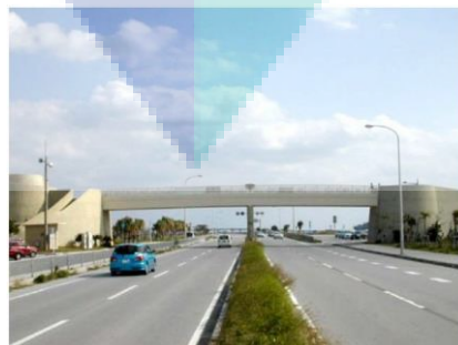
Figure 2.3 Okinawa road park GFRP bridge
