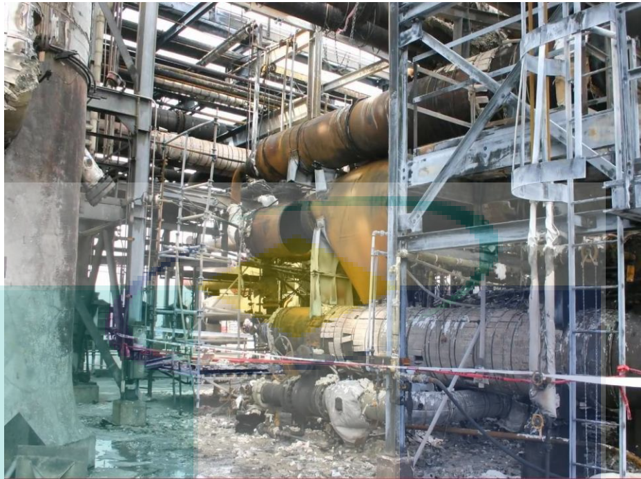
Figure 0.2: Fire and Explosion at Tesoro Anacortes Refinery (John, 2014)
