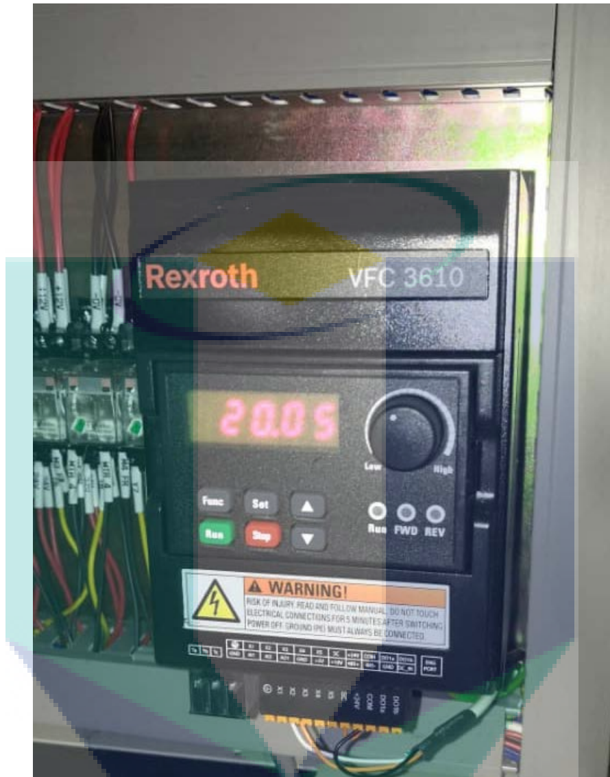
AC Motor Inverter for Motor Speed Control
