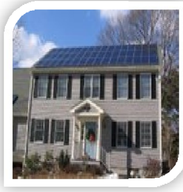
Photovoltaic solar panels on roof.
