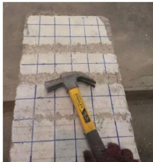
Fig. (8b). The RC beam's surface was roughened.
