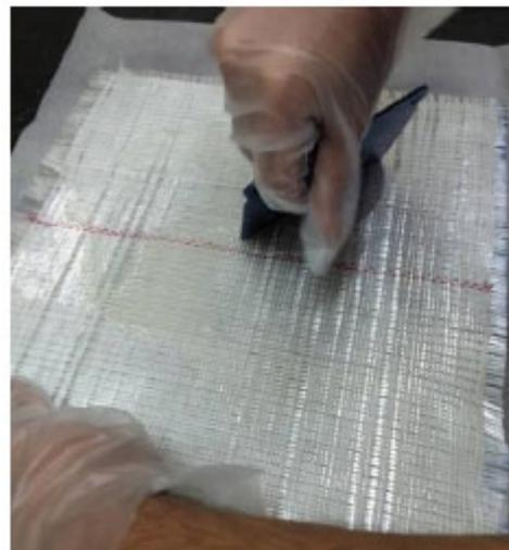
Fig. (3). Spreading the epoxy evenly on the GFRP sheet.
