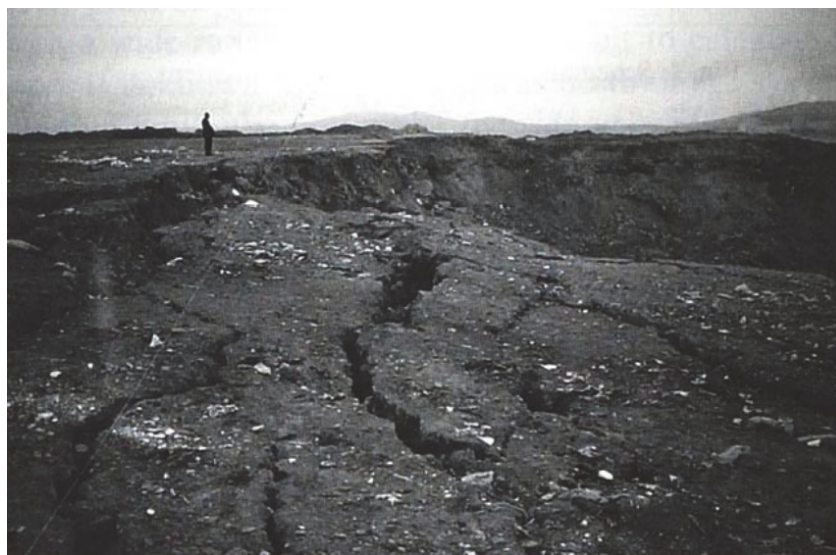
Figure 19: The initial multidirectional tension crack in the cracked zone of the landfill [5].
