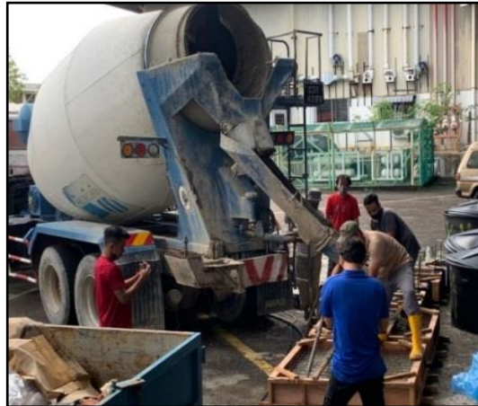
Figure 1. Ready-mixed delivered concrete.
