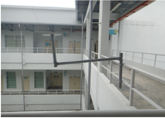
Figure 4. Magnetics antenna to detect EMF
