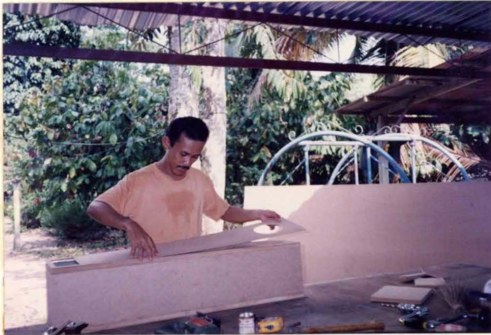
Rajah 3.24: Kerja-kerja penampal papan lapis
