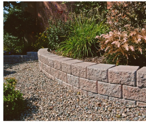
Fig. 16. Wedge blocks at a wall.
