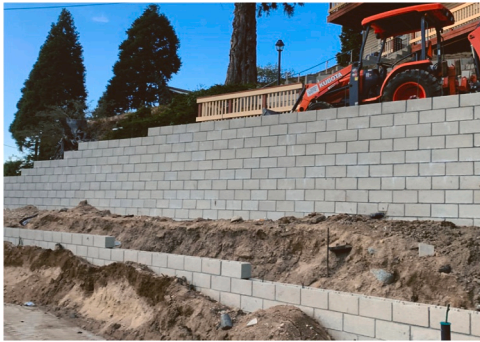
Fig. 9. Gravity retaining wall.
