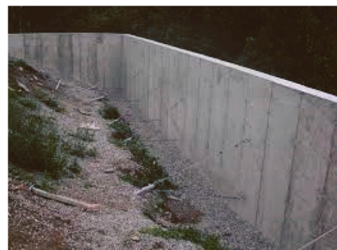
Fig. 13. Cantilever retaining wall.
