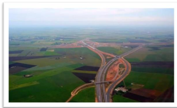
Figure 2.3 Snap with a drone of road construction surveying
